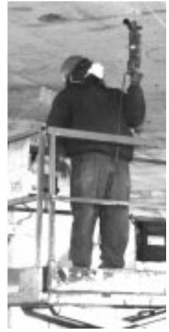
Willie Pittman, IBEW Local 103, drills into a concrete ceiling.
