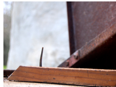
Figure 22. Nail protruding from wood.
