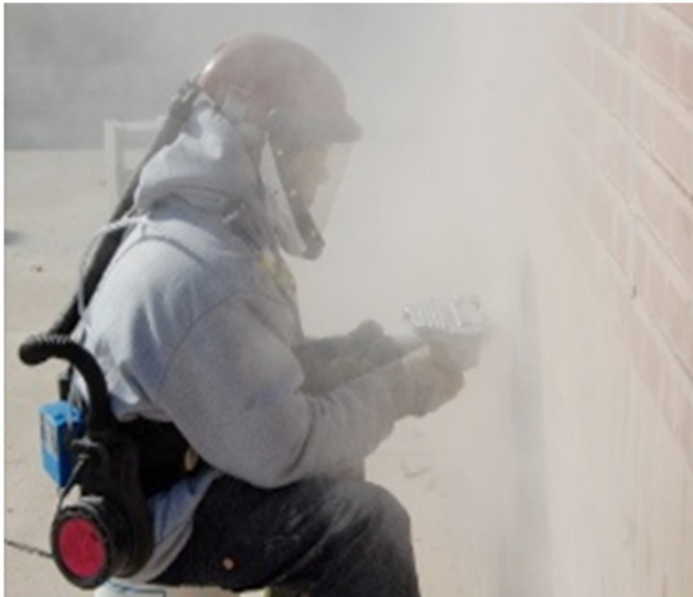
Figure 39. Tuck-pointing without controls
