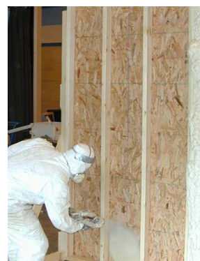
Figure 36. JobCorp student using a soy-based spray foam.
