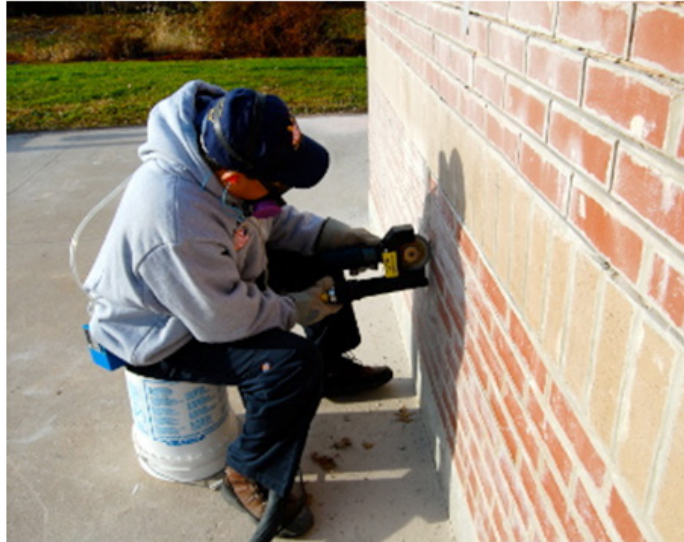
Figure 40. Tuck-pointing with controls
