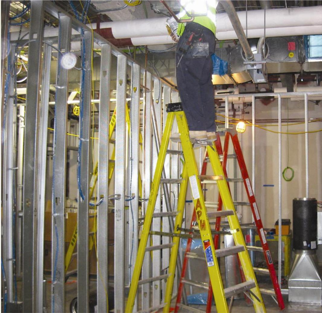
Unsafe posture. Worker should be on a lower rung; a taller ladder is needed.
