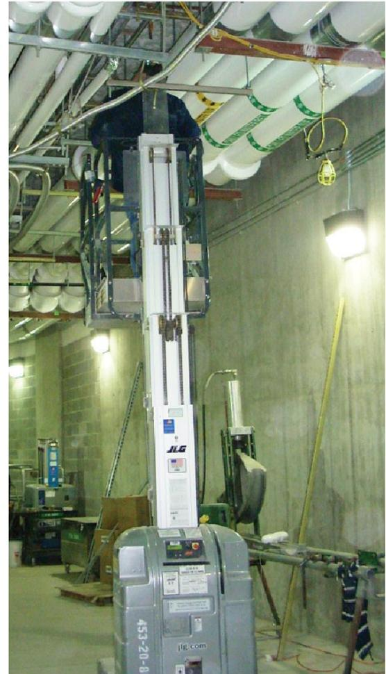
The lift on the right allows a worker to reach heights while providing a safe working platform and small footprint in the hallway compared to the very tall step ladders on the left that are still not tall enough for the workers to safely reach their job tasks.
