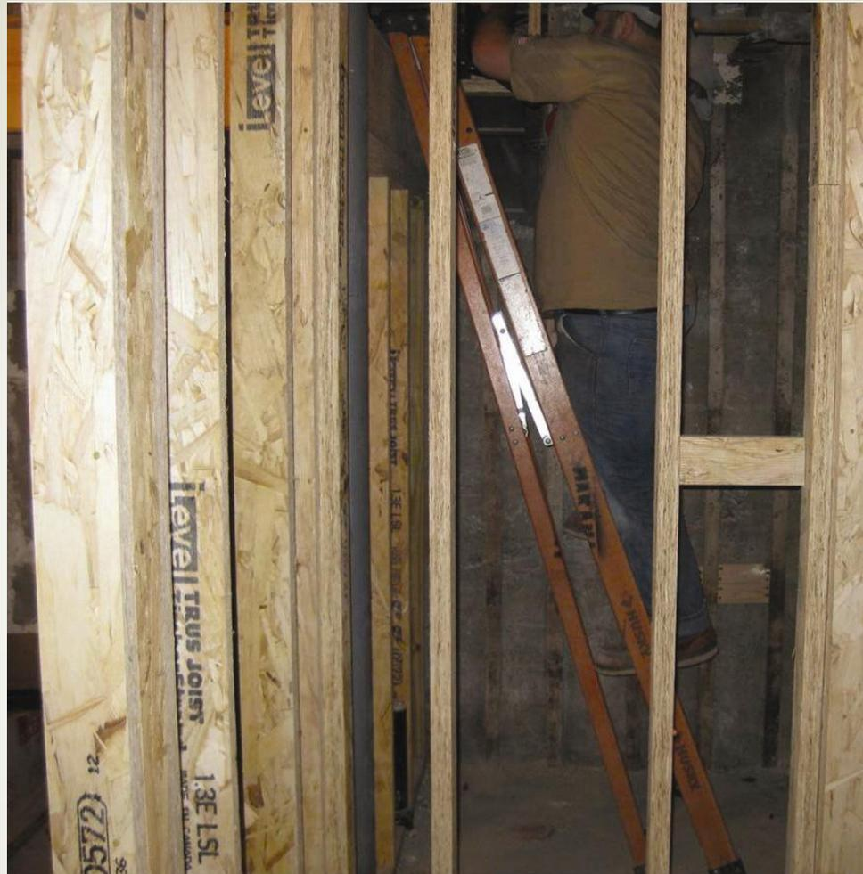
Ladder is placed incorrectly. Ladder should be extended out with its spreaders locked. If the work area is too small, an alternative should be used.
