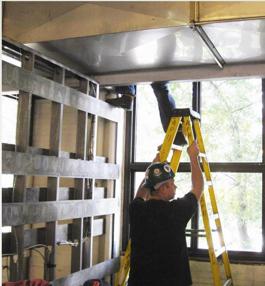
Unsafe posture. Worker should be facing the ladder and on a lower rung. A taller ladder facing the opposite direction may be necessary.
