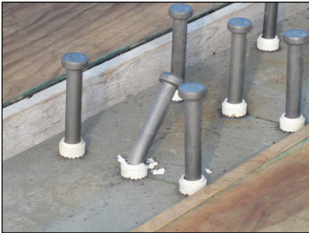
Figure 1: Welded shear stud connectors with ceramic ferrules during bridge construction.
