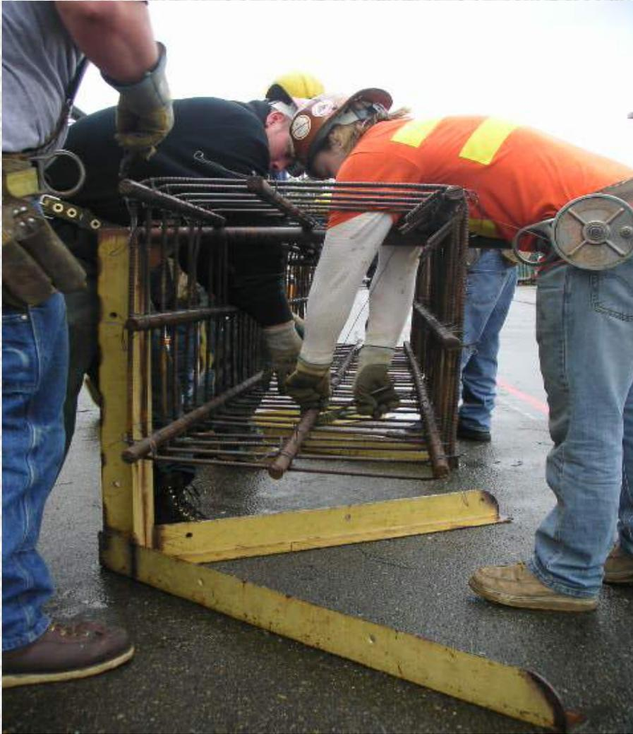
Simple **support stands** can be used to raise material and equipment from ground level, making lifting and working easier and increasing the weight that can be lifted.
