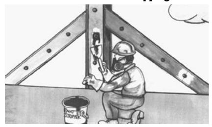
Stripper is applied to steel surface and left in place for 1-24 hours. Paint and stripper are scraped off and residues are wiped away. Some strippers require neutralization.
