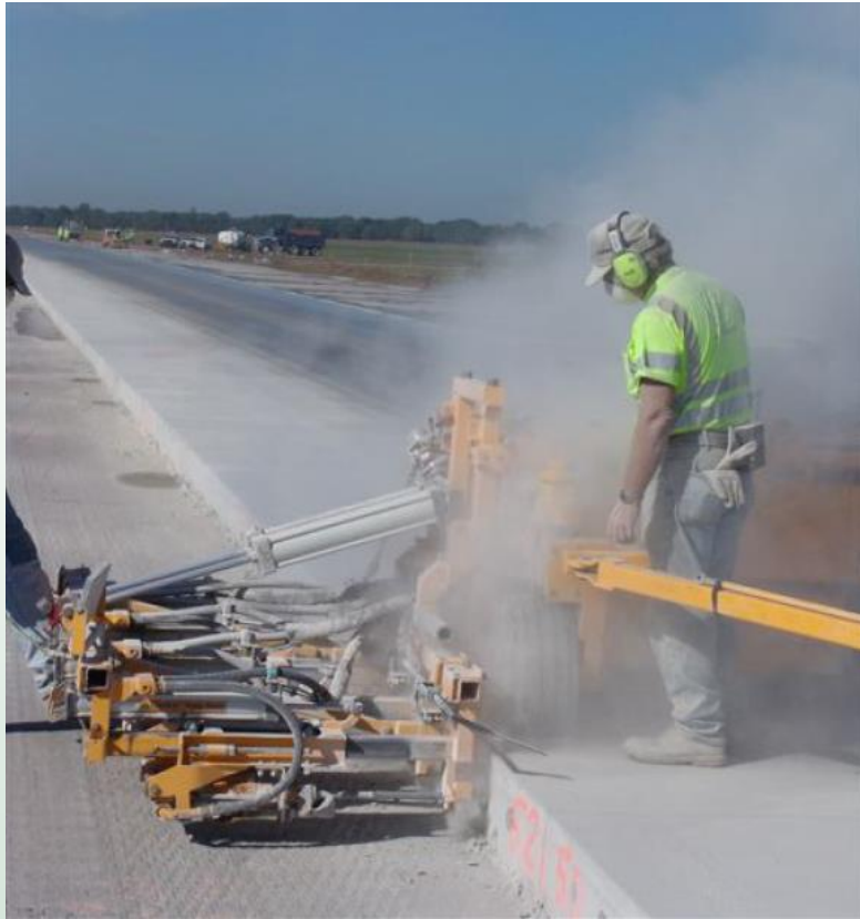
Without Local Exhaust Ventilation
