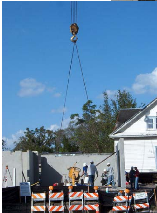
Modular, insulated wall units
