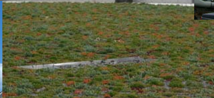
Rooftop rain garden
