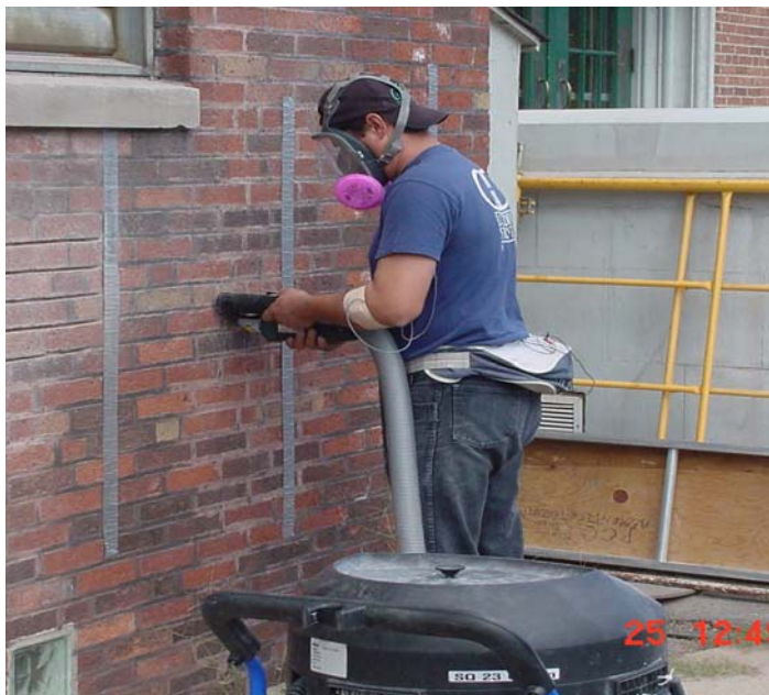
Figure 1. A vacuum cleaner exhausts air from a hood mounted on a grinder used for mortar removal.
