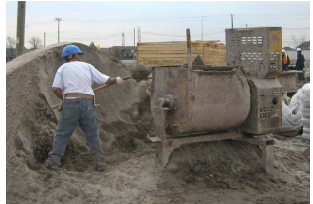
Traditional method of transporting grouting using buckets.
