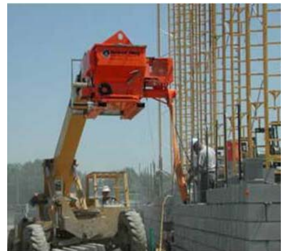
Grout delivery system
