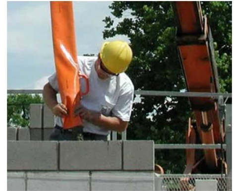
Filling the blocks
